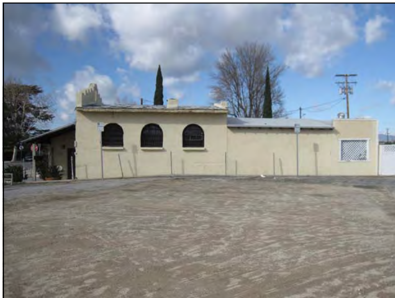
Figure 4: Old Newhall Jail, south elevation, view north (CA, 2010).
