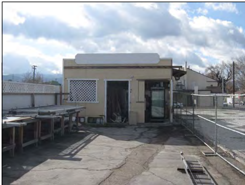
Figure 6: Old Newhall Jail, east, view west (CA, 2010).
