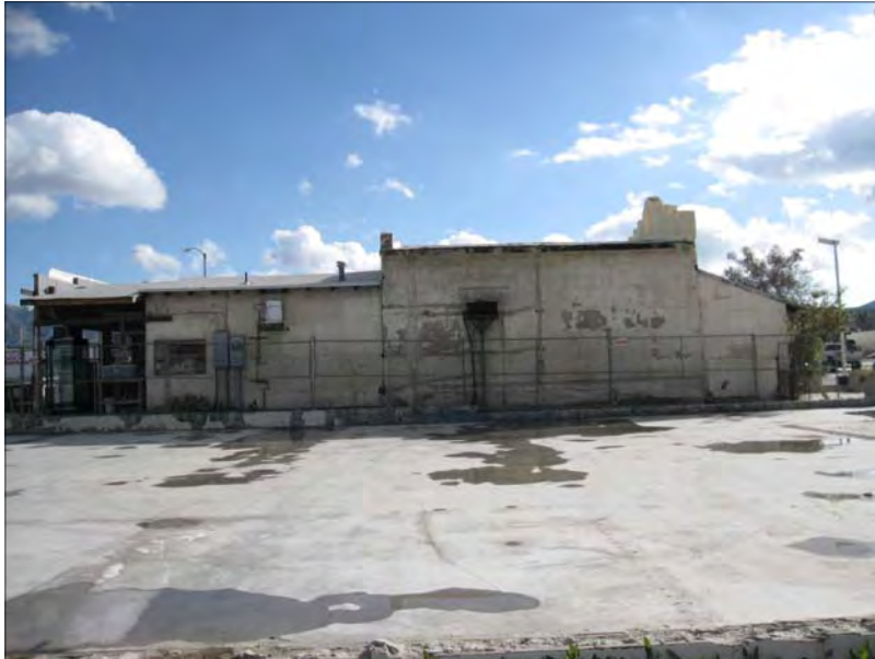
Figure 5: Old Newhall Jail, north elevation, view south (CA, 2010).
