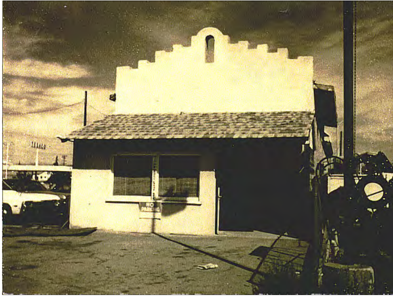
Figure 7: Old Newhall Jail, east elevation, view west, 1960s (Santa Clarita Valley Historical Society).
